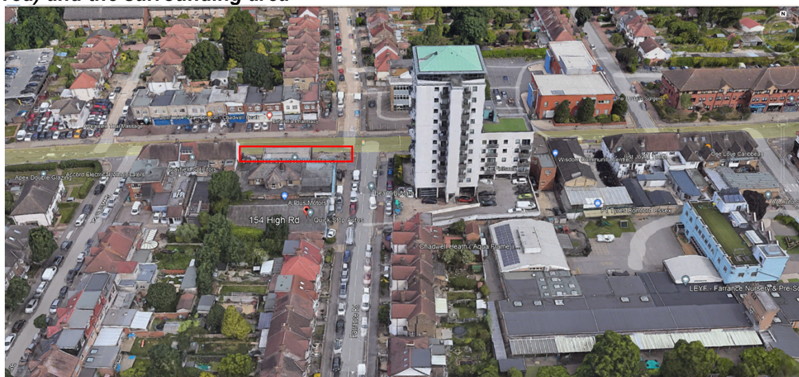
Figure 1: Google Earth screenshot of aerial view of the application site (marked red) and the surrounding area
